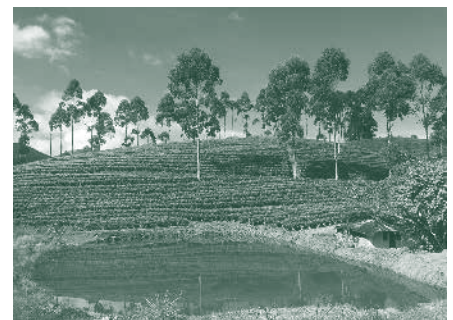
Rain Water Harvesting - Alton Estate
